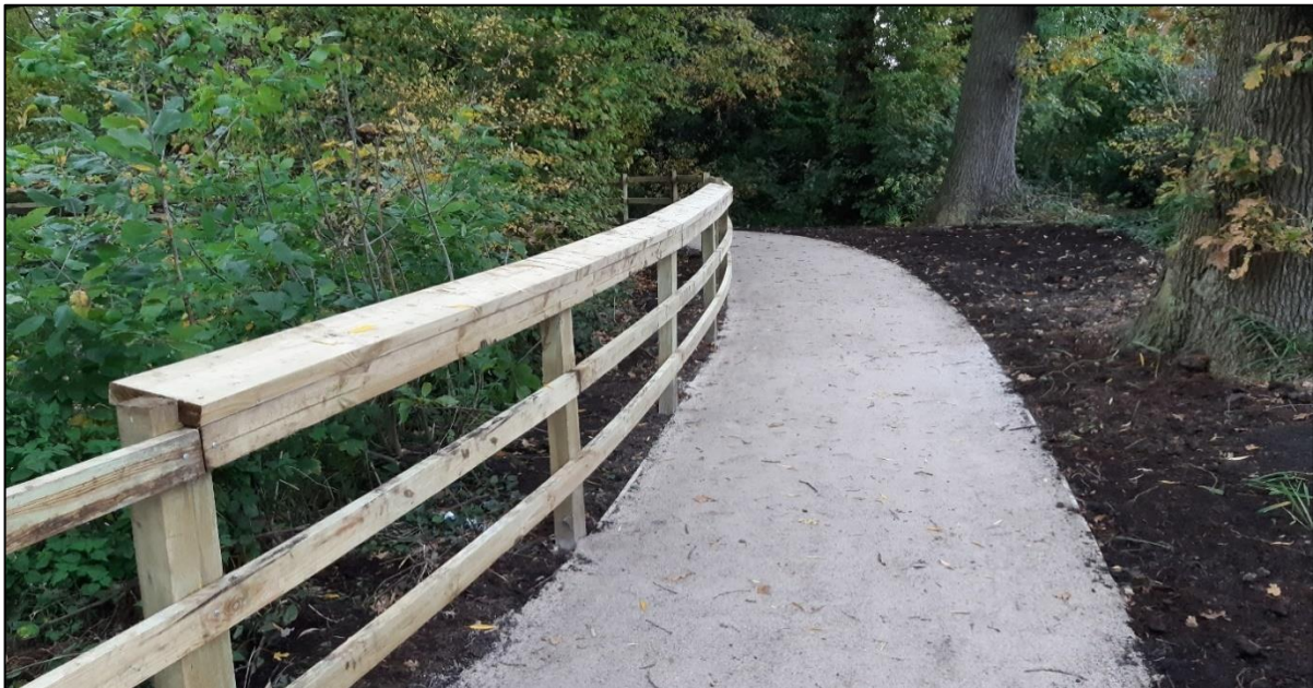
Tarn Wood, Penwortham - Replacement of a woodchip track with a stone path and improvements to the pond overflow drainage system funded by S106 green infrastructure contributions.
